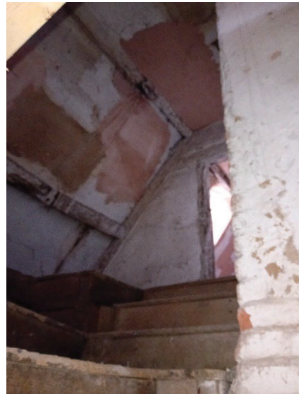
Photo 7: B1 converted loft space – no PRFs present
